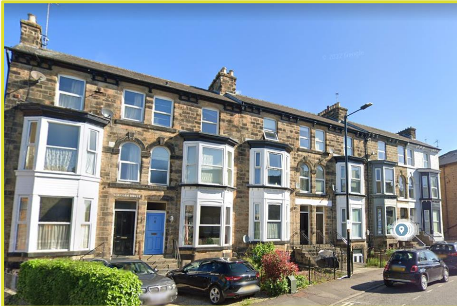
Flats in the W. Knaresborough zone
