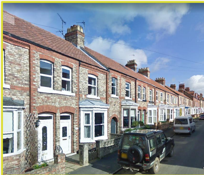
Terrace dwellings in the Malton to Sand Hutton Zone
