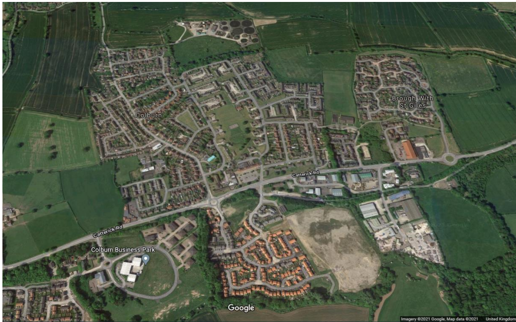
Figure 115: Aerial image taken from Google Maps of Colburn Waste Water Treatment Works and the surrounding area.
